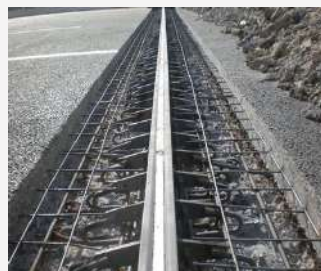
Strip seal expansion joints are installed in highway
