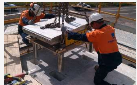
The installation of pot bearing.
