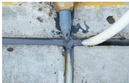
Black single component polyurethane water-swelling sealant in construction joints.
