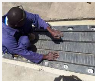
Rubber bridge expansion joint installed in end of bridge
