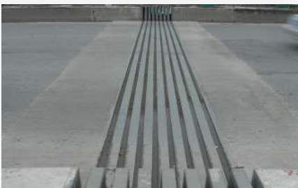
The large-span bridge is being built with multiple-gap expansion joints
