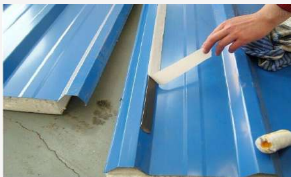
Color steel plate splicing
