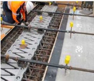
The bridge is being built with finger expansion joints
