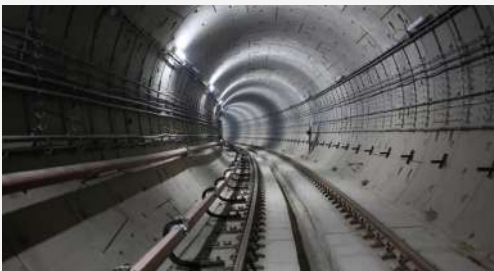
Splicing of tunnel waterproof board.
