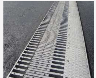
Finger expansion joints are installed in connection of bridges
