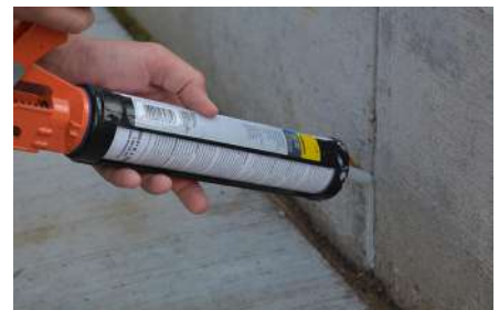
White single component polyurethane water-swelling sealant in wall seam.
