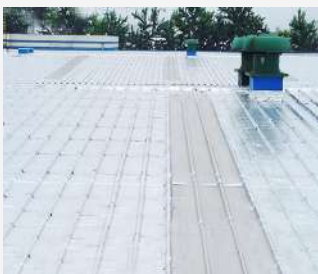
Roof waterproofing
