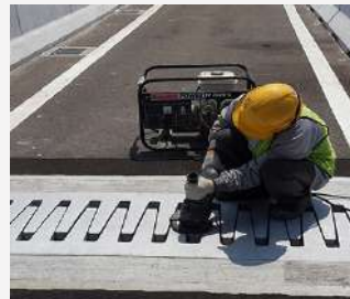
Finger expansion joints are used in end of bridge
