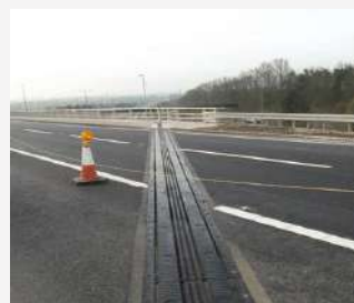
Rubber bridge expansion joint is used in flyover
