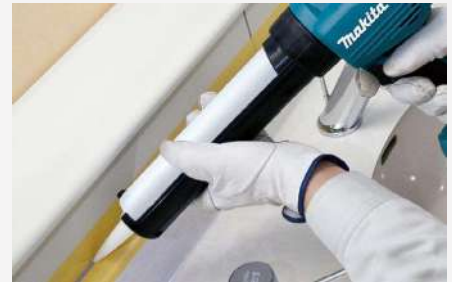
Neutral silicone structural adhesive sealant is used in bathroom.
