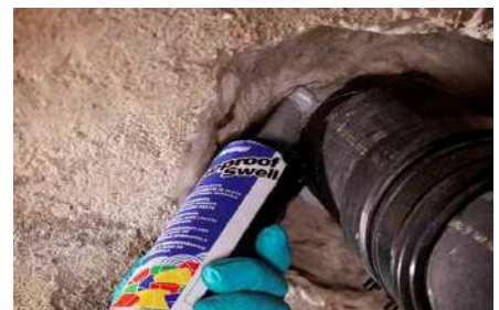
Black single component polyurethane water-swelling sealant used in pipe trench.
