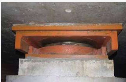
Guided sliding pot bearing is used for bridge.
