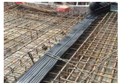
EVA waterstop is used in foundation to prevent seepage.
