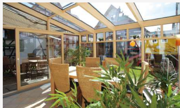
Sun room waterproof sealing
