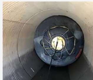
Industrial pipeline cleaning
