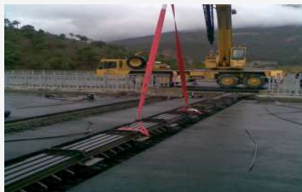
A large-span bridge that has completed with multiple-gap expansion joints
