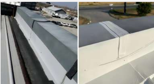
The sealing of the joint of the gutter.
