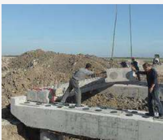
Round laminated bearing pad in bridge construction.
