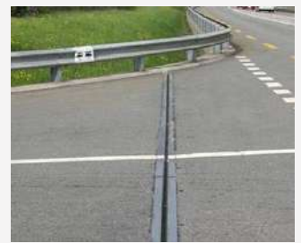
Strip seal expansion joints are installed in highway
