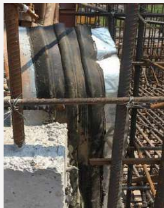
Steel edge waterstop for foundation waterstop.
