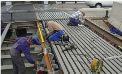
The large-span bridge is being built with multiple-gap expansion joints
