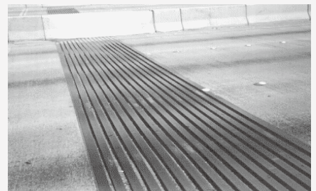
Multiple-gap expansion joints are being installed in bridge
