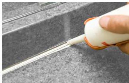
White single component polyurethane water-swelling sealant in ground seam.
