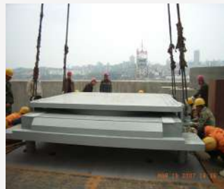
Construction site of bridge spherical bearing.
