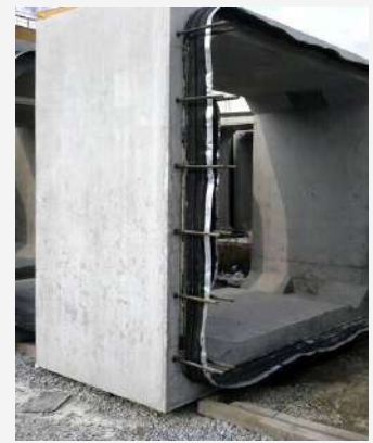
Steel edge waterstop for boundary waterproof.
