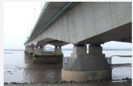
Rectangular PTFE bearing pads on right bridge.
