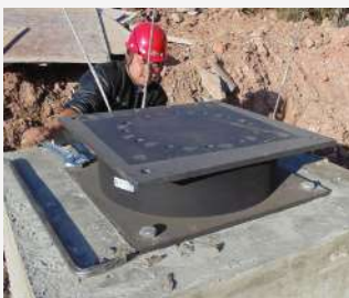
Lead rubber bearing fixation.
