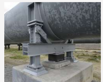
Lead rubber bearing for steel bridge construction.
