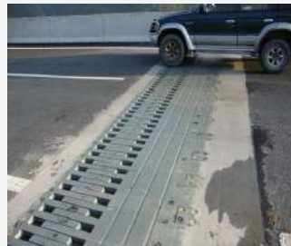
A bridge that has been built with finger expansion joints
