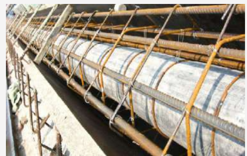
Rubber inflated culvert balloon placed into the rebar cage
