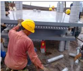
Construction site of structure spherical bearing.
