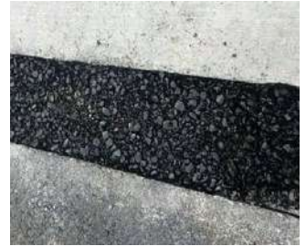
Asphaltic plug joint is used in end of bridge
