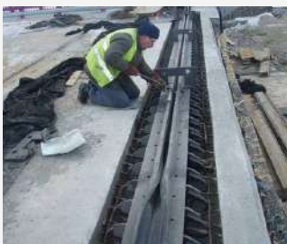
Strip seal expansion joints installed in end of bridge
