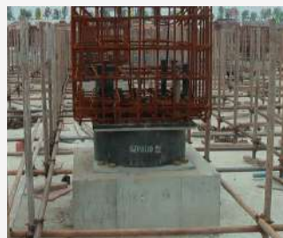
Lead rubber bearing in the construction site.
