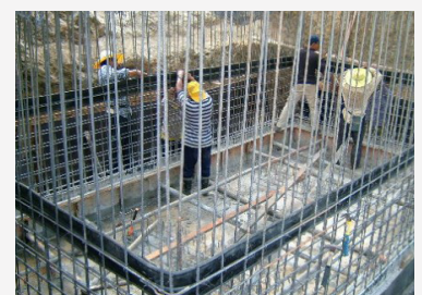
EVA waterstop is used in retaining walls
